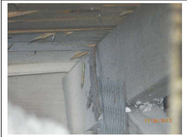
Strap wrapped with one nail
