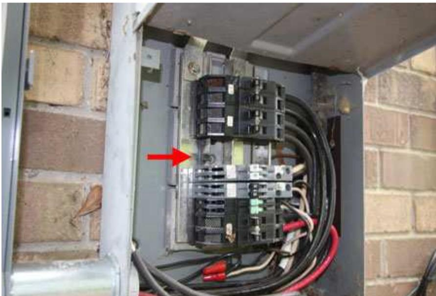
Zinsco Panel Box with Cover Removed (F09-026).
